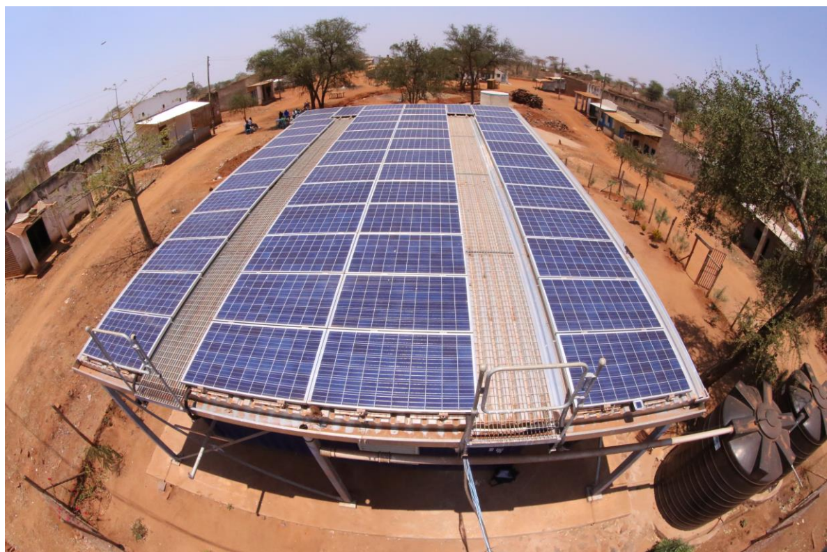
Figure 2. PV system in Kitonyoni trading centre where the modules were installed on a canopy that provides shading for the community as well as harvesting rainwater ( 2 \times 10,000 l storage tanks, front right of image).
