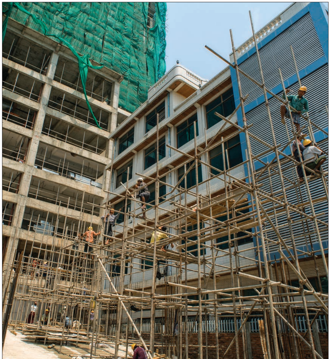
Workers assemble a scaffolding at a construction site in Yangon
