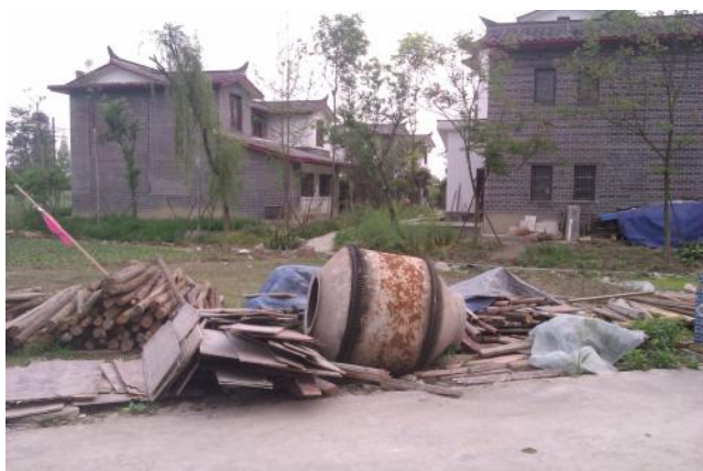
Fig. 8. Mr. Chen’s construction equipment and materials on the public green. (Source: Author’s photo.) (For interpretation of the references to color in this figure legend, the reader is referred to the web version of this article.)
