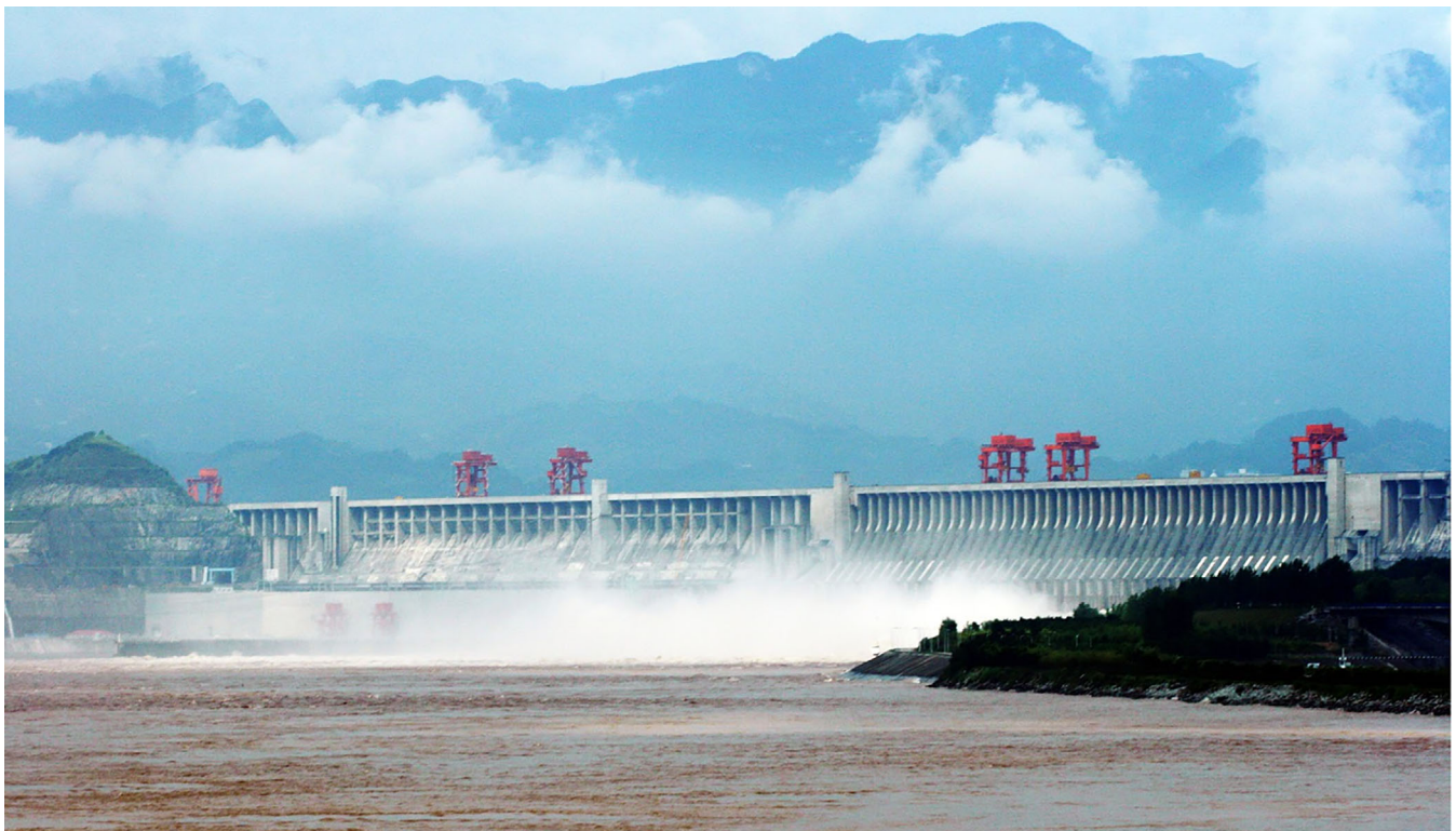
FIGURE 3 The Three Gorges Dam Reservoir approached maximum storage in August 2020 after receiving near-continuous inflow of 75,000 m 3 /s for about 1/3 a day (CGTN, 2020). The high flows were the result of flooding in the upper reaches of the Yangtze River. The widespread flooding was described as the worst in about 40 years. Extreme discharges on the Yangtze at Yichang of ~71,000 m 3 /s were recorded in 1896 and 1981. Part of the motivation to build this dam was the flood of 1954 where 33,000 people died, many perishing from disease. Photo: 10724842 Kun Yang | Dreamstime.com
