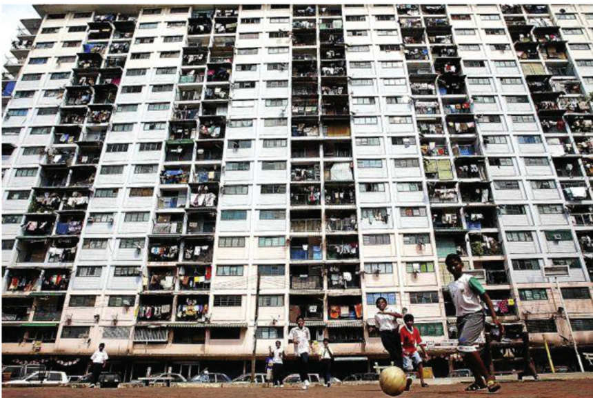
Figure 3. The Pekeliling Flats opened in the 1960s in Kuala Lumpur (The Star 2013).
