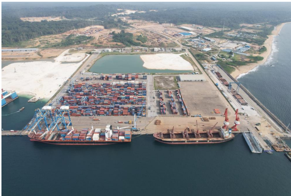
Figure 4-7 Kribi Deepwater Port Container Terminal
