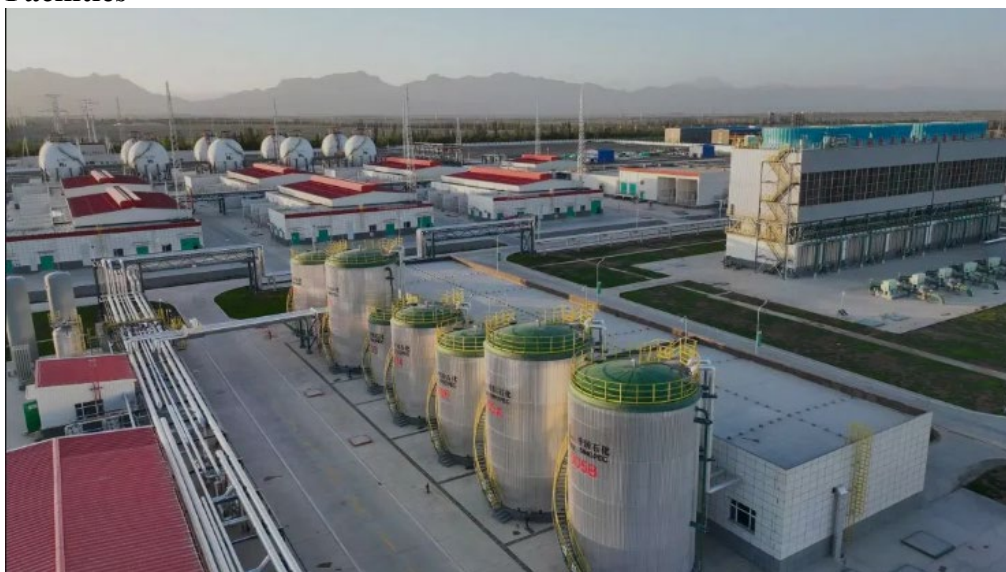
Fig. 6.3.3 Xinjiang Kuqa Green Hydrogen Demonstration Project On-site Facilities
