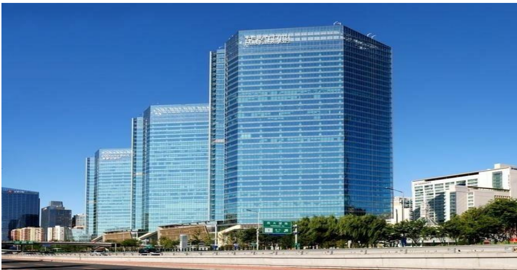
Fig. 5-8 Huamao Office Building
