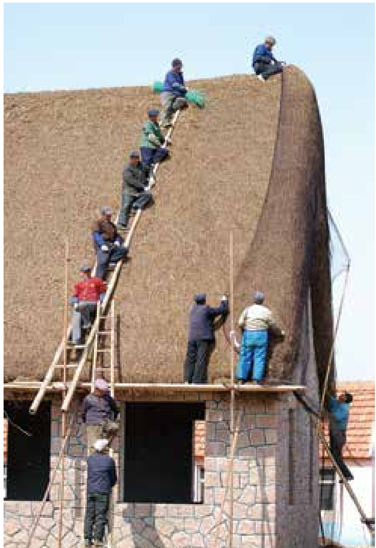
Lu Jia, 2011. Building of a seaweed house. The average age of a seaweed house builder is over 60—the building technique will be lost if younger generations do not practise and pass on this skill.
