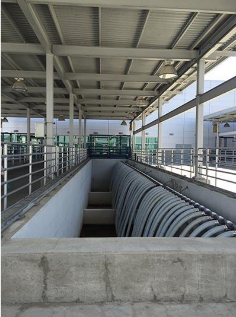
Image: GWRS microfiltration facilities. Photo by author.
