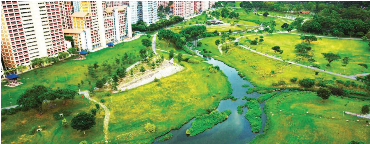
Bird-eye view of the rejuvenated Bishan – Ang Mo Kio Park. The area features a meandering waterway flanked by park land that serves as a floodplain during wet weather and as a recreational space during dry weather. (Source: PUB, Singapore’s National Water Agency)
