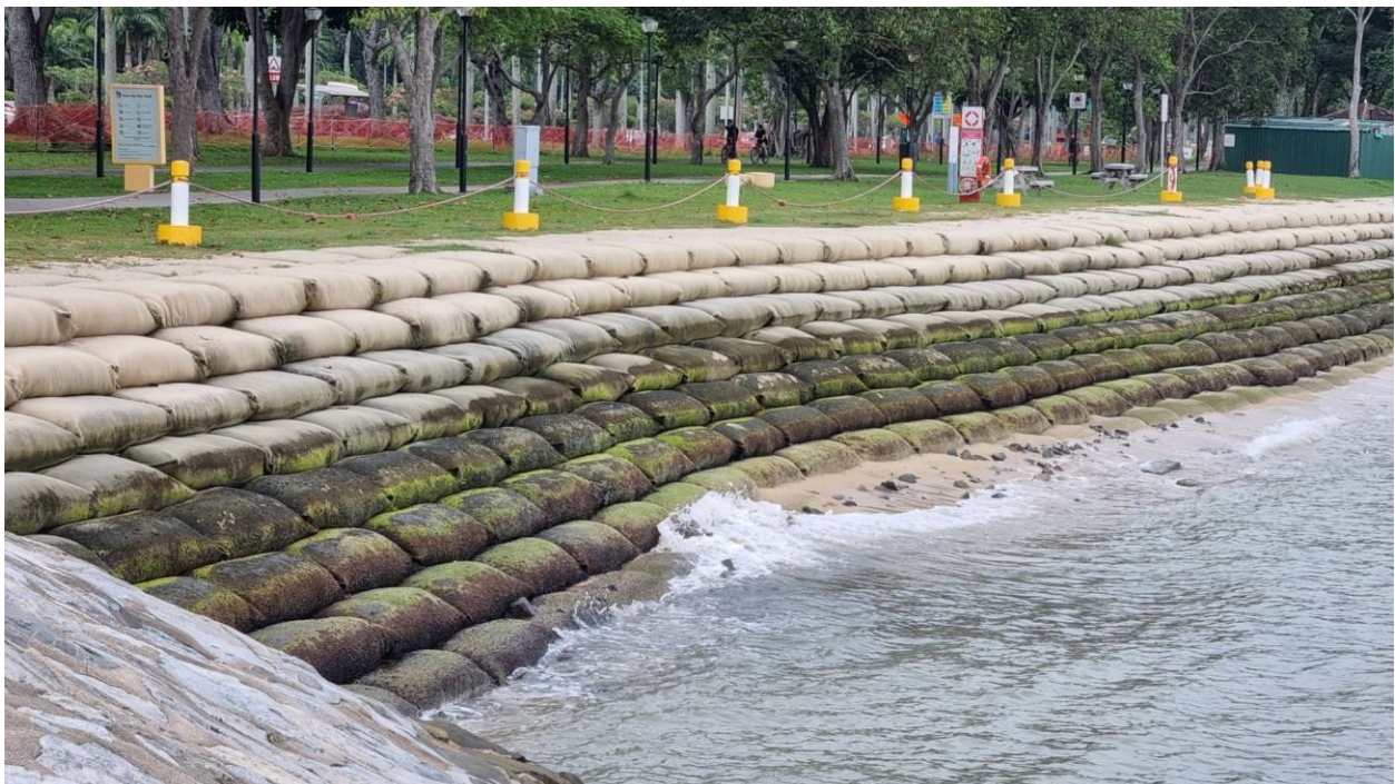
Sandbags a storey high placed along the coastline from Bedok Jetty to the East Coast Lagoon (Photo source: TheHomeGround Asia )
