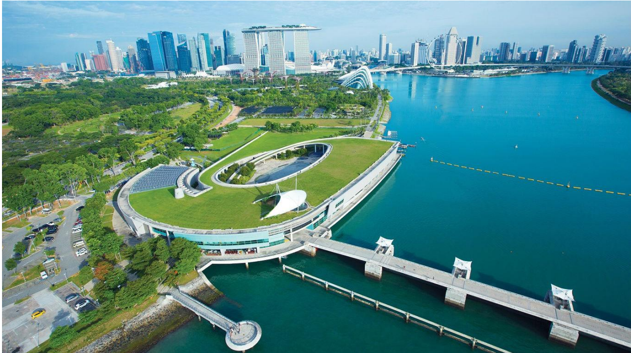
Marina Barrage serves three purposes: a source of water supply, flood control, and a venue for lifestyle attraction. (Source: PUB Singapore's National Water Agency)
