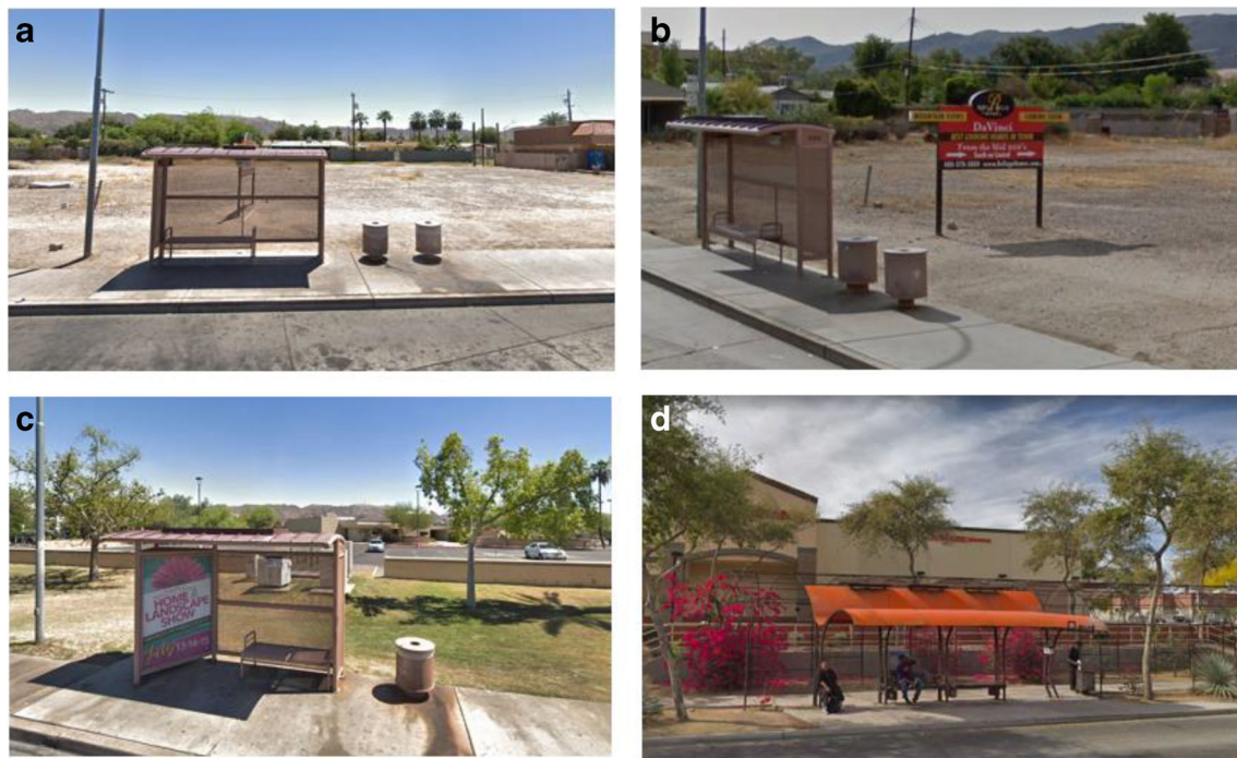
Fig. 1 Types of bus stops and design attributes examined during the field campaign between June 6 and July 27, 2018. a Standard bus stop shelter. b Standard bus stop shelter with a standalone advertising sign used for
