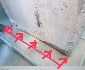
Toilet plaster work wear and tear due to constant moisture. Sealant was observed to be missing around the edges. (Before)
