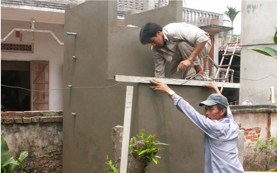
Locals were trained to build, operate and maintain their own household arsenic removal water filters.
