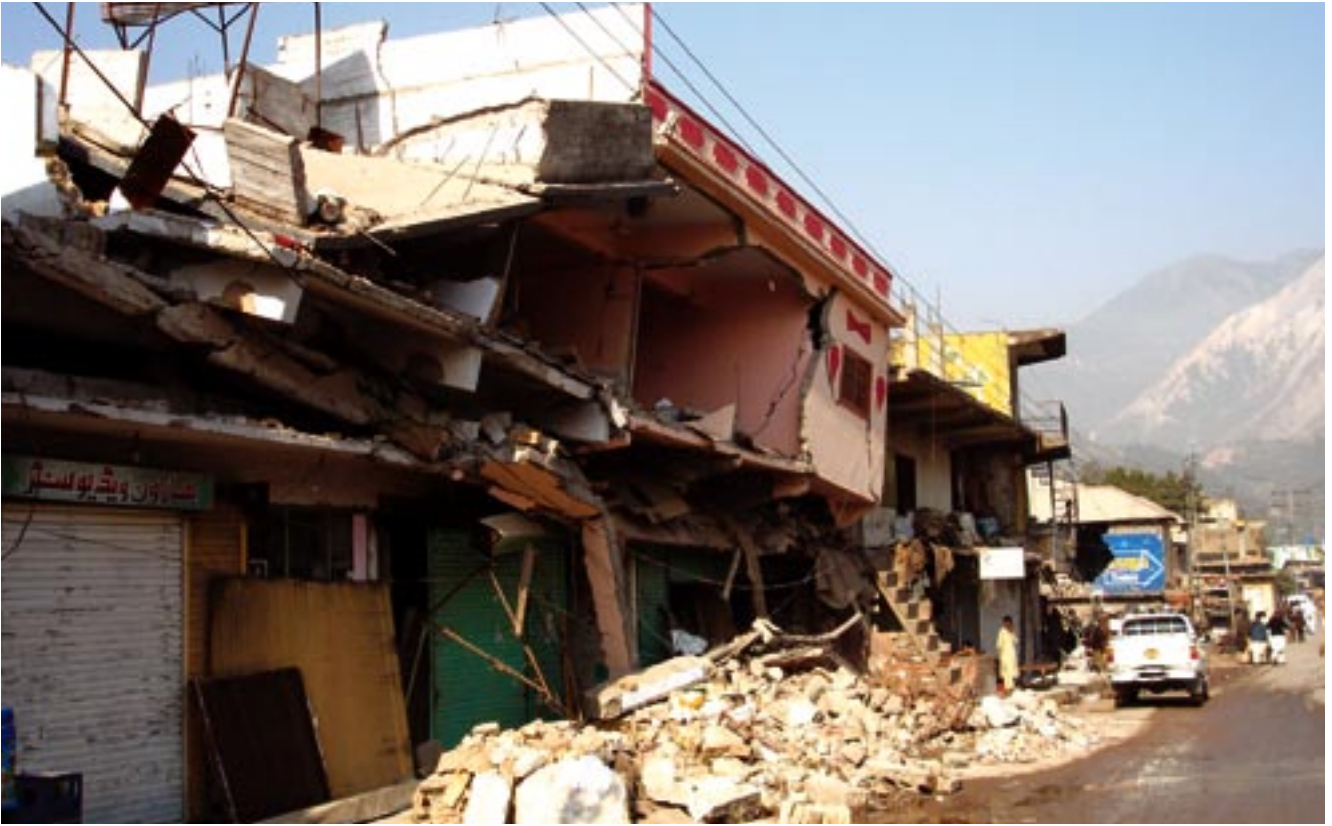
Earthquake damaged city, Muzaffarabad, Pakistan Earthquake 2005
